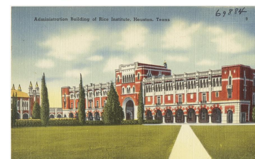
Rice University coat of arms and administrative building
